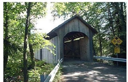
After the bridge, bear right at the first fork and go 0.8 miles to the Morgan Bridge, another 60-foot queenpost built in 1877. It features some unique reinforcing rods in the trusses and five-foot gable overhangs not found on other queenpost bridges in the county.
