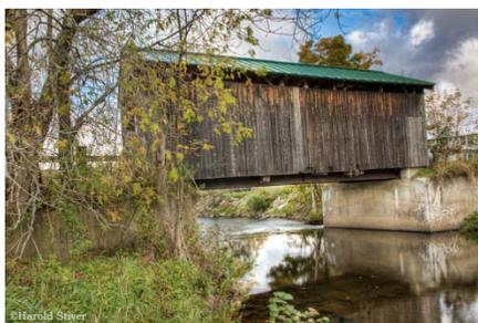
comparatively recent origin, this 45-foot queenpost over the Gihon River was built in 1919, probably as an open bridge, with massive timbers for such a length. Reconstructed in 1960, the deck is supported by four steel beams and the original stone abutments were replaced with concrete, a good example of historical authenticity bowing to modern requirements.
